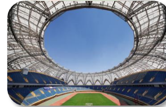
Construction Stadium Roofing
