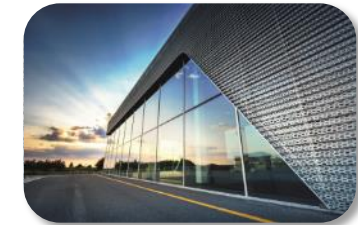
Construction Metal Panel
