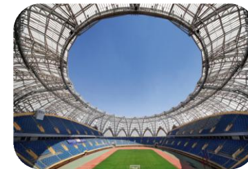
Construction Stadium Roofing
