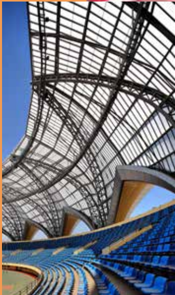
For challenging architecture and futuristic design, polycarbonate can be used as roofing for athletic stadiums, such as here in Beijing, China.
